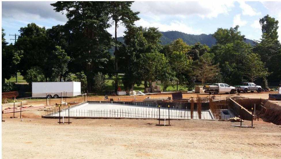
The base of the indoor heated program pool is our first concrete pour.
